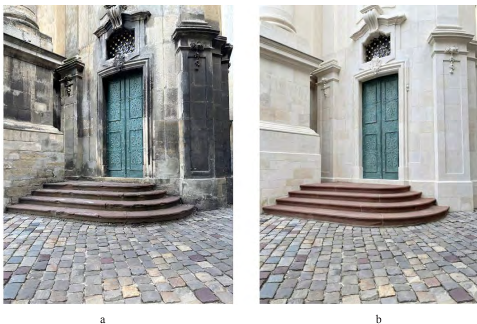
Fig. 1. Portal of the Church of the Most Holy Eucharist in Lviv: (a) present condition; (b) reconstruction of the probable original colouring of the stone
